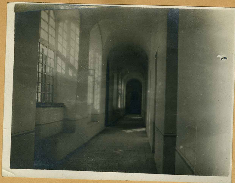
Corridor note windows
